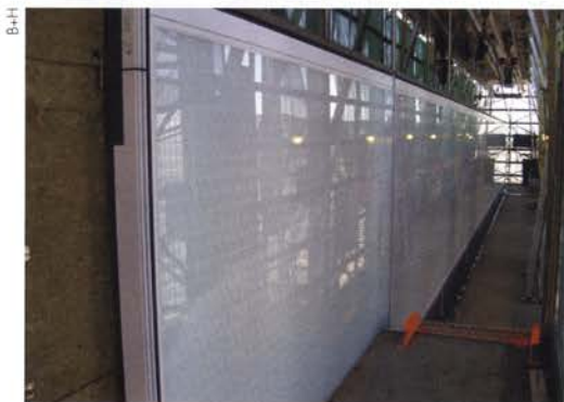
ABOVE, CLOCKWISE FROM TOP LEFT THE ORIGINAL MARBLE CLADDING; THE ORIGINAL SEALANT, INSULATION AND STONE PANELS ARE REMOVED AND REPLACED WITH THE NEW CLADDING ASSEMBLY; THE NEW UNITIZED PANELS ARE INSTALLED; THE GLASS PANELS AS THEY ARE LOADED INTO POSITION. BELOW, LEFT TO RIGHT AN AERIAL VIEW OF FIRST CANADIAN PLACE WHEN IT OPENED IN 1975; AN ELEVATION OF THE ORIGINAL MARBLE PANELS. BOTTOM, LEFT TO RIGHT THE FIRST OPTION OF THE FRIT PATTERN; A SECOND, DENSER FRIT PATTERN DID NOT RESPOND WELL TO CHANGING LIGHT CONDITIONS; THE FINAL FRIT PATTERN SELECTED FOR THE RECLADDING OF THE BUILDING.
